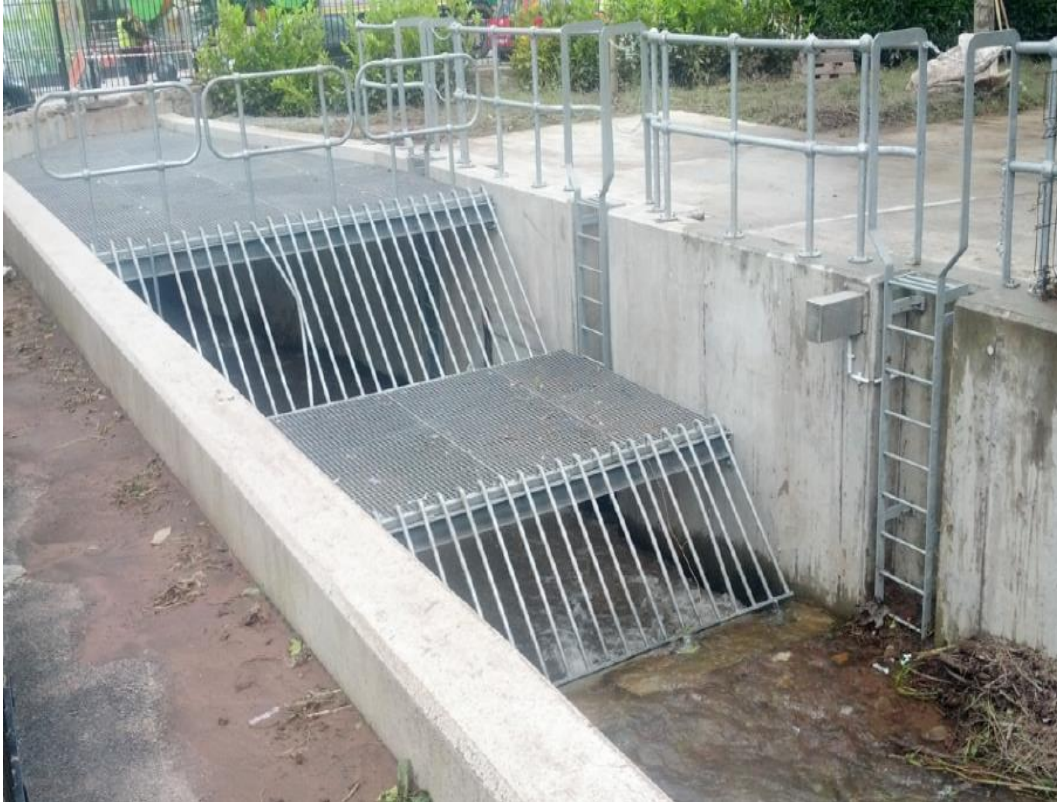
Figure 2.4: Church Road culvert trash screen – normal conditions. Source: OPW
