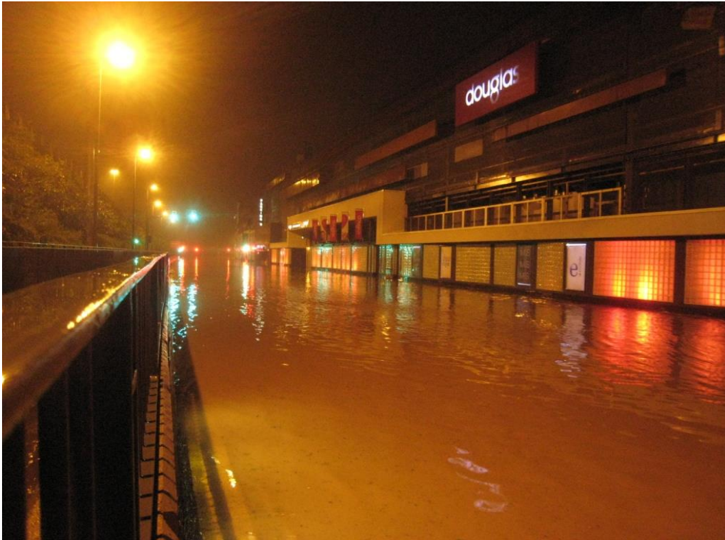
Figure 2.9: Post 2012 flood event outside Douglas Village Shopping Centre. Source: Cork County Council
