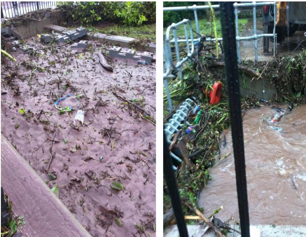
Figure 2.5: Church Road culvert trash screen – post 2012 flood event. Source: OPW
